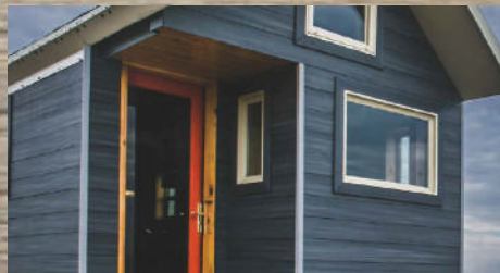
External Facade Claddings
