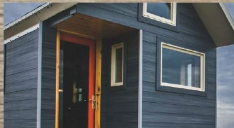
External Facade Claddings
