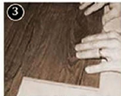
Press down and lock into place
