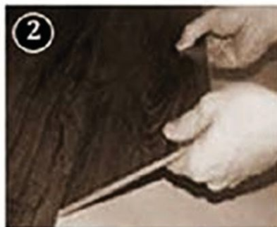
Angle the second plank and align the interlocking strips
