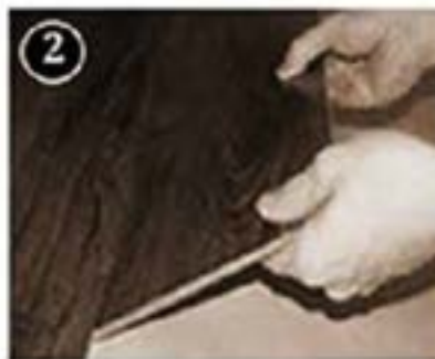
2 Angle the second plank and align the interlocking strips
