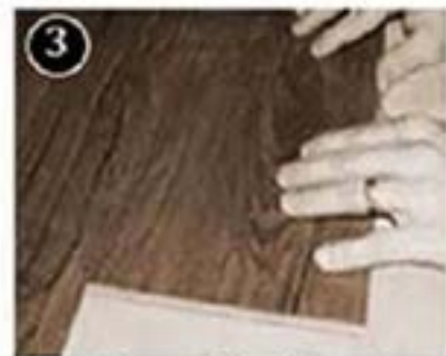
3 Press down and lock into place
