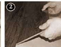
Angle the second plank and align the interlocking strips
