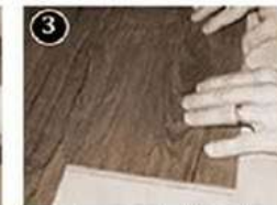
Press down and lock into place
