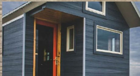
External Facade Claddings
